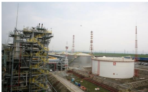
▪ Flare and tank-farm - Start-up 02.2015
