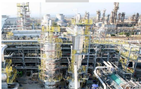
▪ Sulphur recovery unit - Start-up 12.2014 г.
