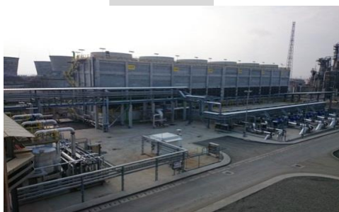
▪ Cooling water - Start-up 11.2014 г.
